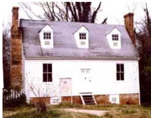
Regrading has protected this masonry foundation wall from excessive damp during its 10-year mothballing. Note the attic and basement vents, temporary stairs, and interpretive sign. Photo: NPS files.
