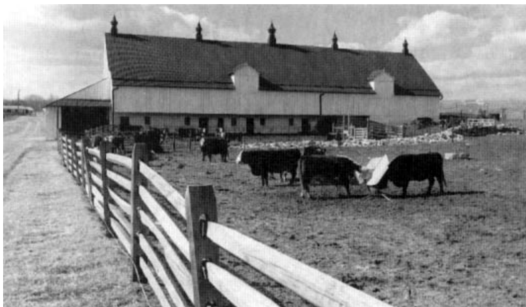
The goal of Preservation is to retain the historic form, materials, and features of the building and its site as they have changed—or evolved—over time. This bank barn was built in the 1820s, then enlarged in 1898 and again in 1914. Today, it continues its role as a working farm structure as a result of sensitive preservation work. This included foundation re-grading; a new gutter system; structural strengthening; and replacement of a severely deteriorated metal roof. Photo: Jack E. Boucher, HABS.
