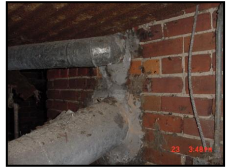
Figure 27: Wrapping on a Pipe
