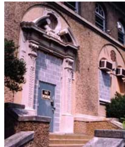
The first floor openings of this historic building have been filled with cinder blocks and the doors, window sash, and frames removed for safe keeping. The security metal door features heavy duty locks. Photo: NPS files.
