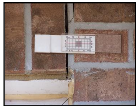
Figure 17: Crack Monitor Gauge
