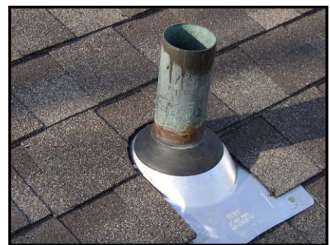
Figure 23: Flashing Around a Vent Pipe
