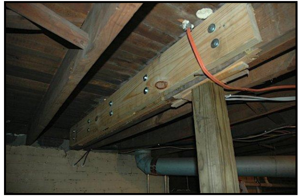
Figure 20: Repaired Rotted Joist
