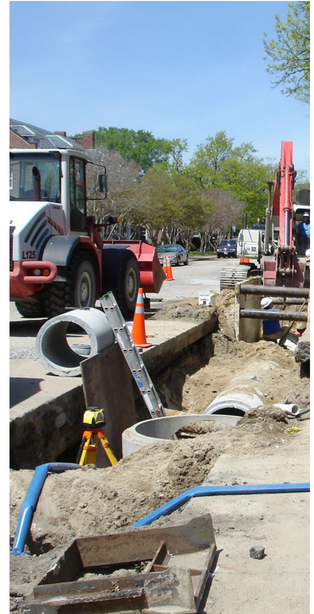
Figure 7B-5: Infrastructure construction on the Fort.
