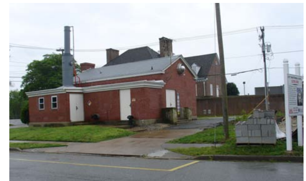
Figure 7B-4: HRSD Willard Avenue Pump Station #225
