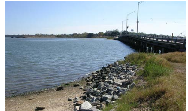
Figure 7B-6: Mugler Bridge.
