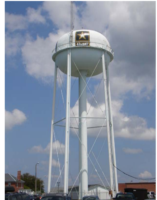
Figure 7B-3: Elevated water storage tank
